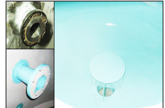
Finished Application of ARC S2
